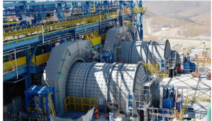
140ktpd throughput design capacity with two SAG and ball mill trains working independently of each other, pebble crusher and regrind circuit.
